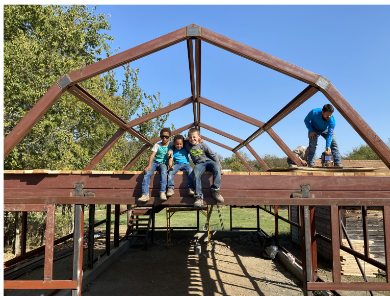
The Aultman family builds a steel barn
